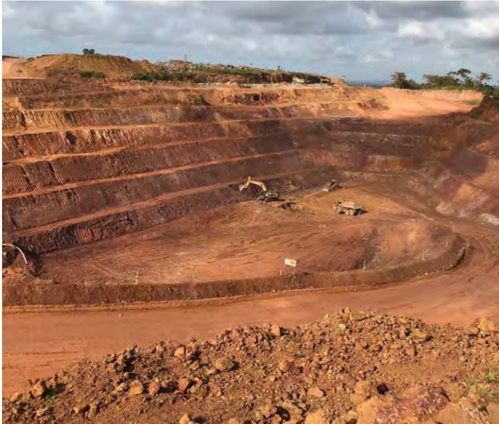
Figure 16-4: Piaba East Wall – August 2021 (Looking West)
